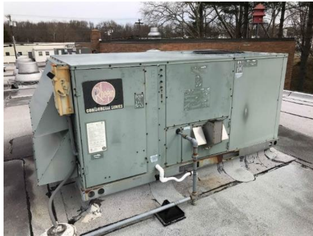
Packaged Roof-Top Unit
