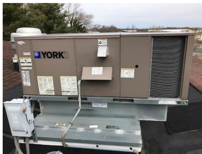
Packaged Roof-Top Unit
